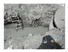
Image H3c. Possible broken pipe; stagnant water with no flow; possible chemical contamination.
